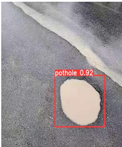
Figure 7: Single road potholes
