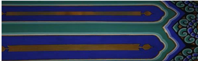
Fig. 2(1) Inner Eaves - pigment layer intact
