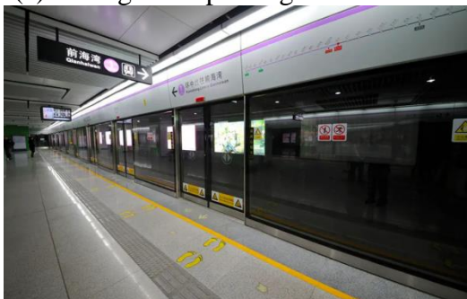
(c) Underground Transportation Facility
