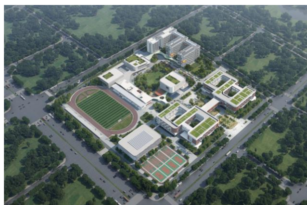
Figure 1: Aerial View (Architectural Design Research Institute of SCUT)
