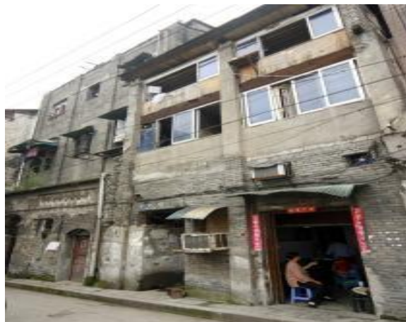
Figure 4: Green infrastructure c human settlements are dilapidated and block
