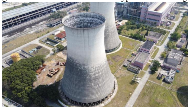
Figure 1: Aerial View of the Reinforced Concrete Hyperbolic Cooling Tower
