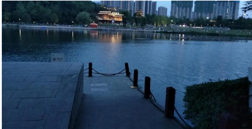
Figure 11: Embankment enclosed by guardrails
